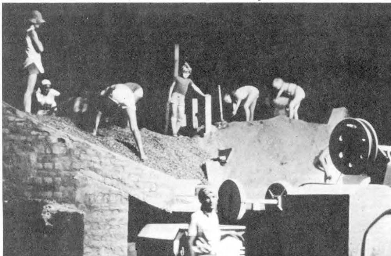
Night concreting for the roof of the inner chamber of the Matrimandir. (Photo by Dominique Darr.)
