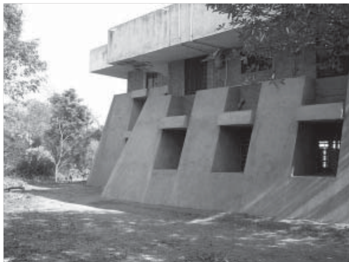
A view of the emerging Pavilion of Tibetan Culture. (Photo courtesy The Pavilion Team)
