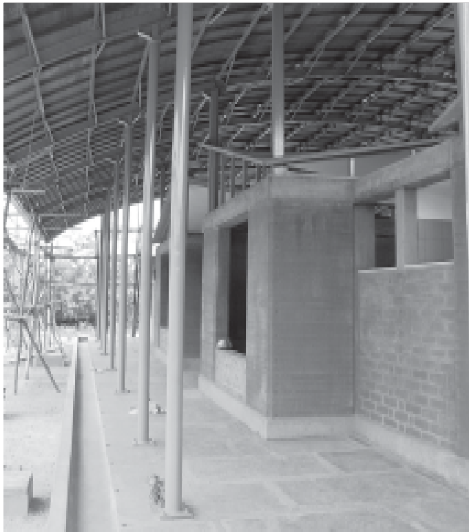
A channel of rainwater protects the building from insects. Steel, ferro-cement, rammed earth and mahogany come together to create a rich palette of local materials. (Photo courtesy Auroville Today)
