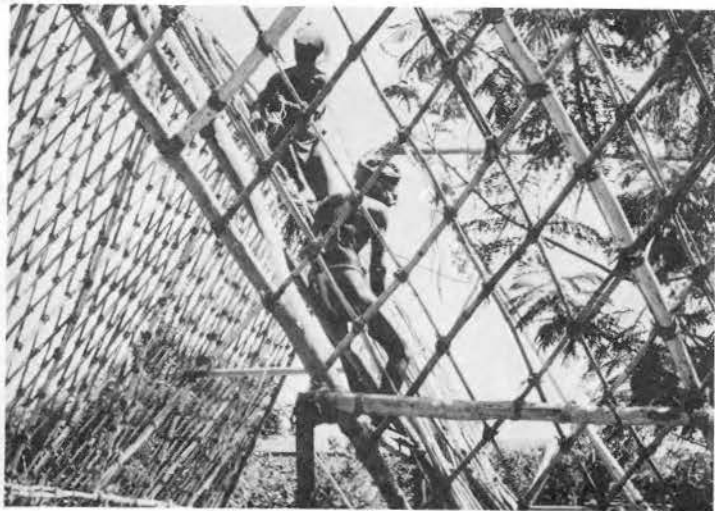
Building a keet and bamboo roof, Auroville.
