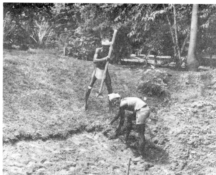
Laying sod and compacting it on a recently constructed earth dam at the Matrimandir Nursery. (Photo by the Nursery.)
